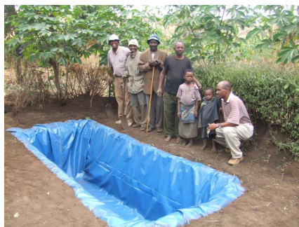
JANI helped ten communities build 61 water storage hafirs to provide irrigation for kitchen gardens in the dry season
